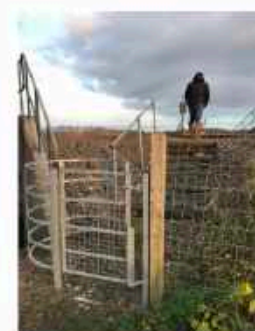
Gate over railway track
