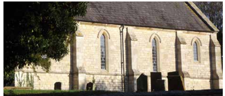
Figure 28: Grade II Church of the Holy Cross, Kirkby Green.
