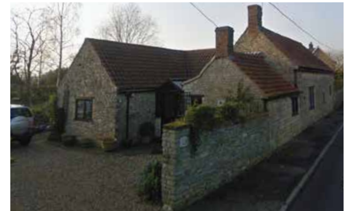
Figure 110: Facade articulated with well proportioned opening.
