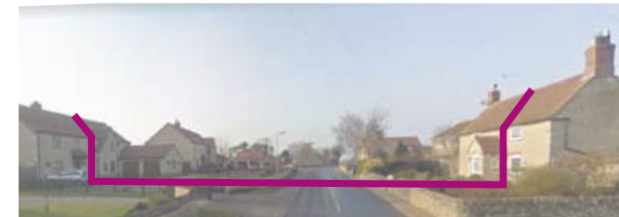
Figure 57: Example of height to width ratio of 1:6, which gives a less sense of enclosure.
