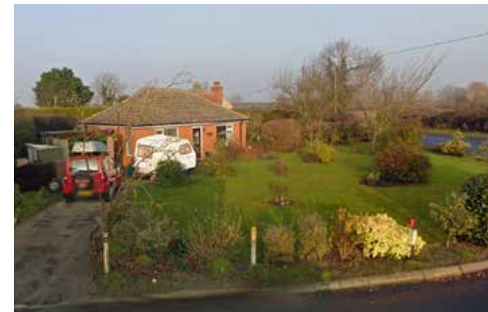
Figure 61: Corner building with windows on the main street.
