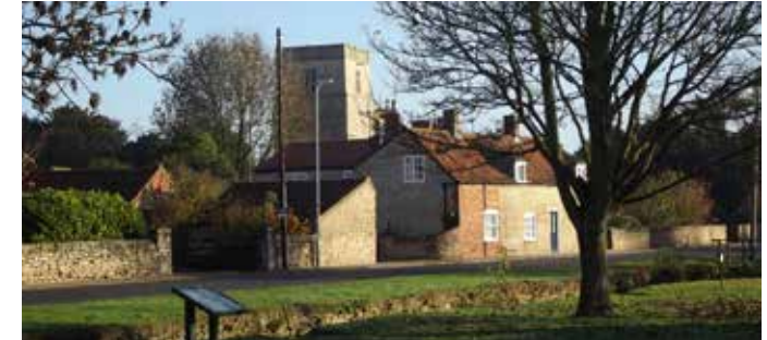
Figure 1: View of Grade II* listed Church of the Holy Cross in Scopwick.
