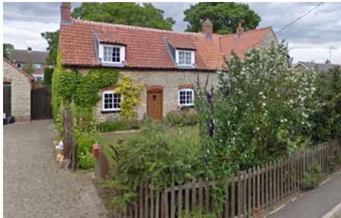
Figure 108: Windows and dormers spaced evenly along the building elevation.
