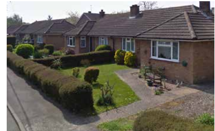
Figure 103: Bungalows at rural edge of the village with large front gardens which allow more daylight.
