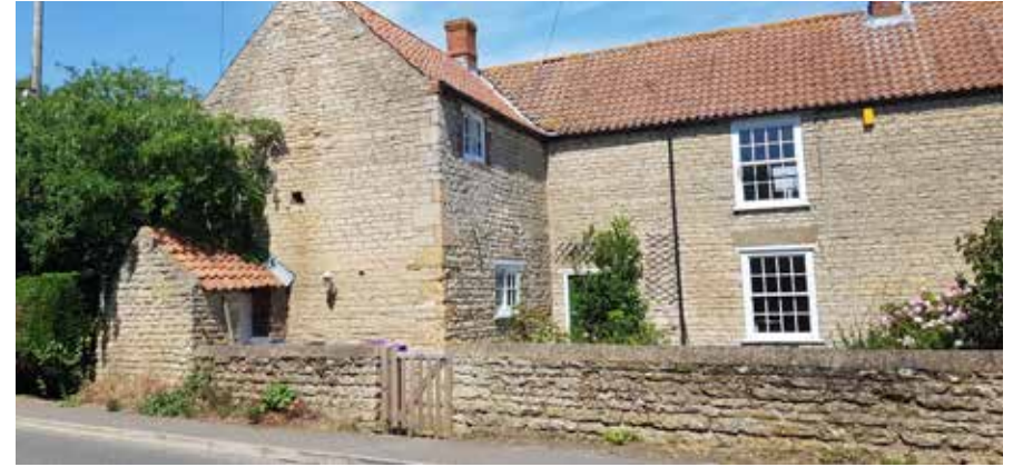
Figure 25: Grade II listed 97-103 Main Street, Scopwick.
