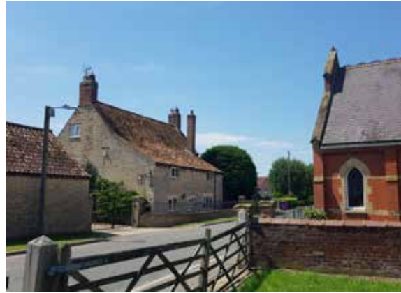
Figure 24: Scopwick Methodist Church.
