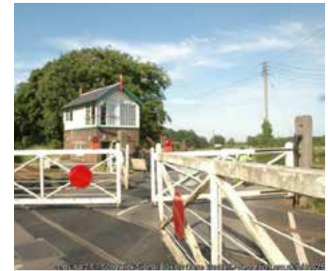
Figure 10: Level crossing in Kirkby Green.
