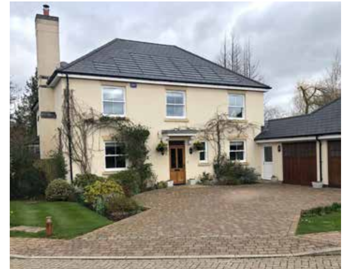
Figure 76: Use of shingle-like solar panels on a slate roof, with the design and colour of the solar panels matching those of the slate tiles.
