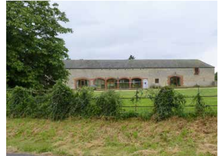
Figure 30: Grade II listed two-storey barn at The Manor House, Kirkby Green. Source © Alan Murray-Rust (cc-by-sa/2.0).
