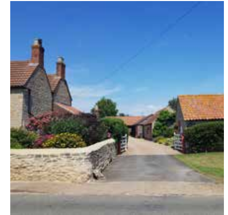
Figure 27: Limestone wall, Kirkby Green.
