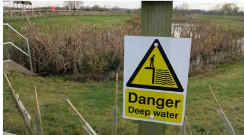
Figure 81: Attenuation ponds and detention basins must be integrated into the green space strategy and designed with safe public access in mind so that they do not necessitate fencing. Designs similar to the facility in this picture must be avoided because they are dangerous and have unattractive fencing.
